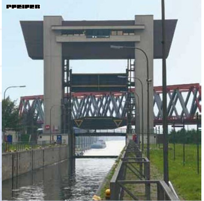
Lock systems: Ropes raise and lower the lock gates
