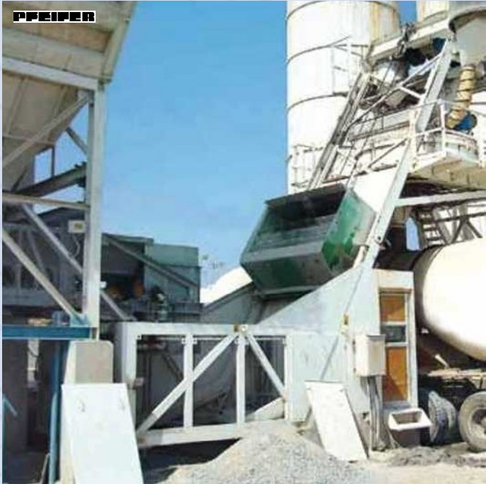
Mixing facilities: Ropes move the feed bucket
