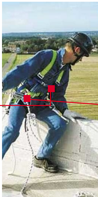
Positioning lanyard EN 354 without energy absorber, to keep distance to the fall edge, or running arrester with fixable rope shortener
