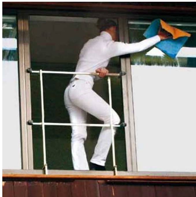
Window fall protection equipment
